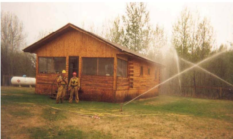
*Figure 9.4. Sprinkler deployment (Rapid Fire and Rescue Inc.).*
